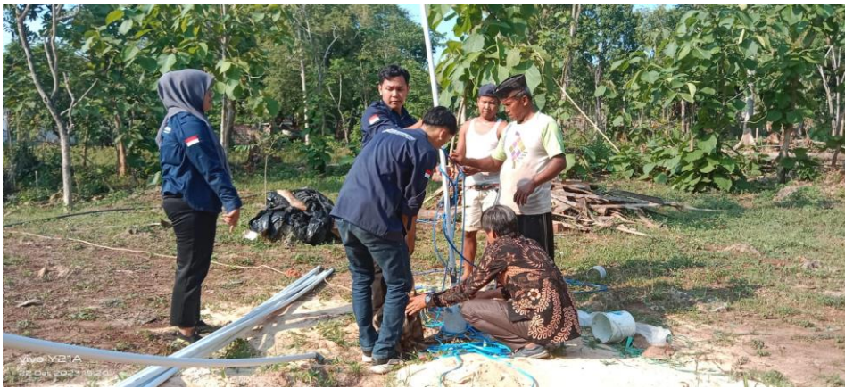
Figure 1. Solar Power Water Pump Install in Ellak Daya, Sumenep
