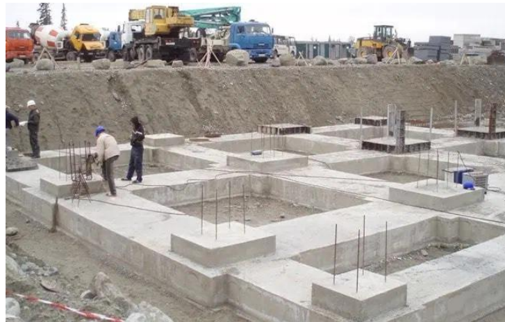
Figure 1. Building Foundation in Construction
