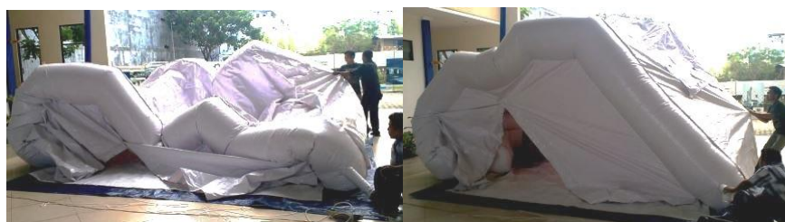
Figure 2. Process Setting-Up Air inflated Structure (Source: Setiawan, M. Ikhsan et.al , 2015 (a))
